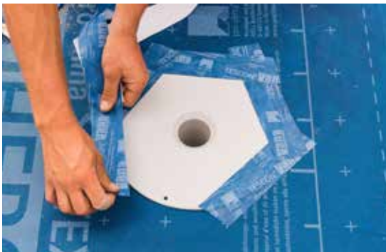
For creating seals between surface-drainage gullies and SOLITEX ADHERO.
