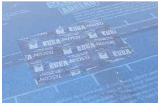
For sealing damaged areas on membranes.
