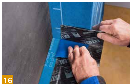
EXTONSEAL ENCORS Waterproof sealing adhesive tape with high adhesion
