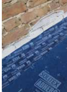
For joints to adjacent building components such as adjacent walls made of masonry, concrete, timber and wood-based panels.
